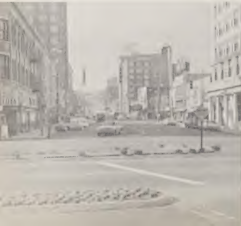
Montgomery Street from the north side of Court Square in 1962. (left)
